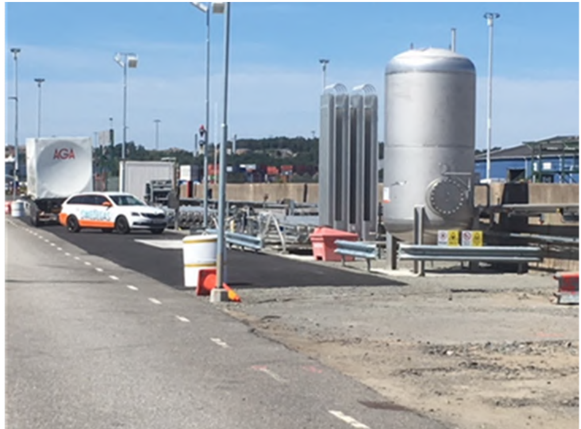
Knock out drum 10m 3 & Vaporizer
